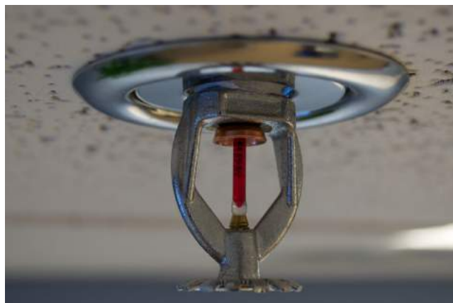
Exposed Fire Suppression Sprinkler
